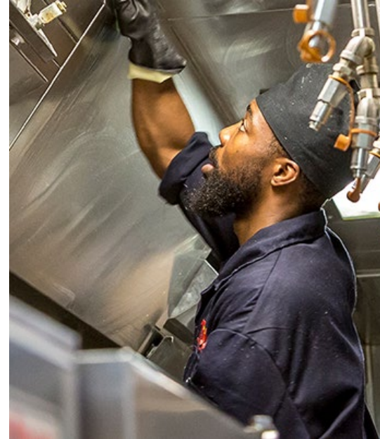
Duct and ventilation cleaning
